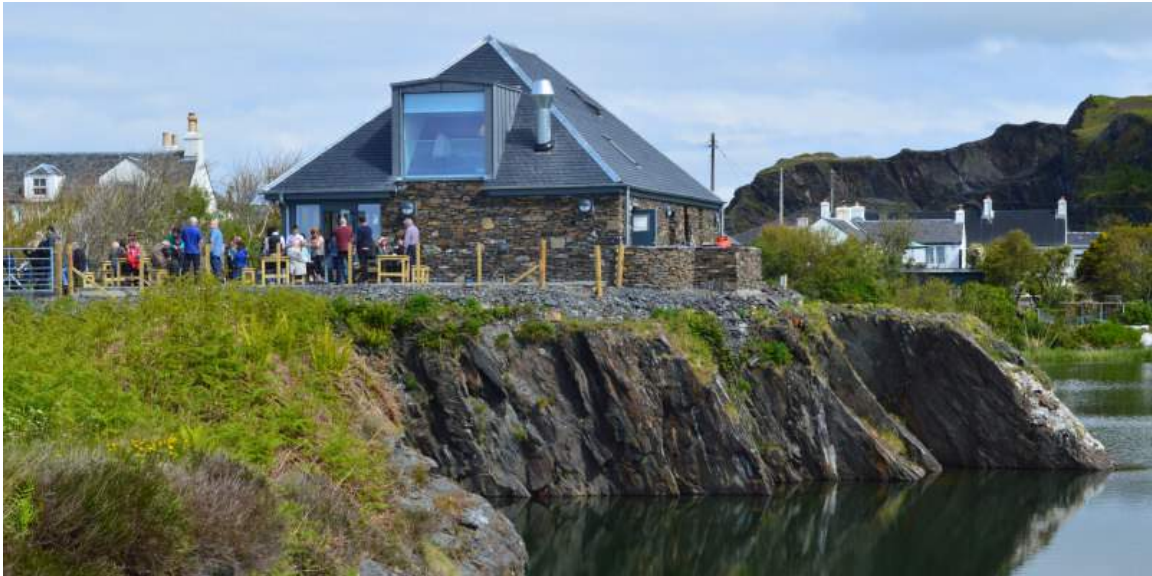
Atlantic Islands Centre showing quarry pond alongside used as heat source for the heat pump system. The slate cladding to the walls of the building conceals an insulated double wall construction inside, while the roof is insulated with over 200 mm thickness of insulating panels
